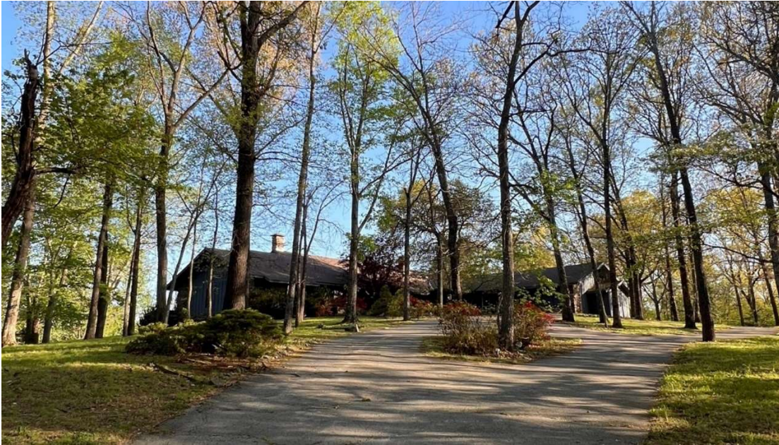
Image 1. Character of structure and existing internal drive and parking area
