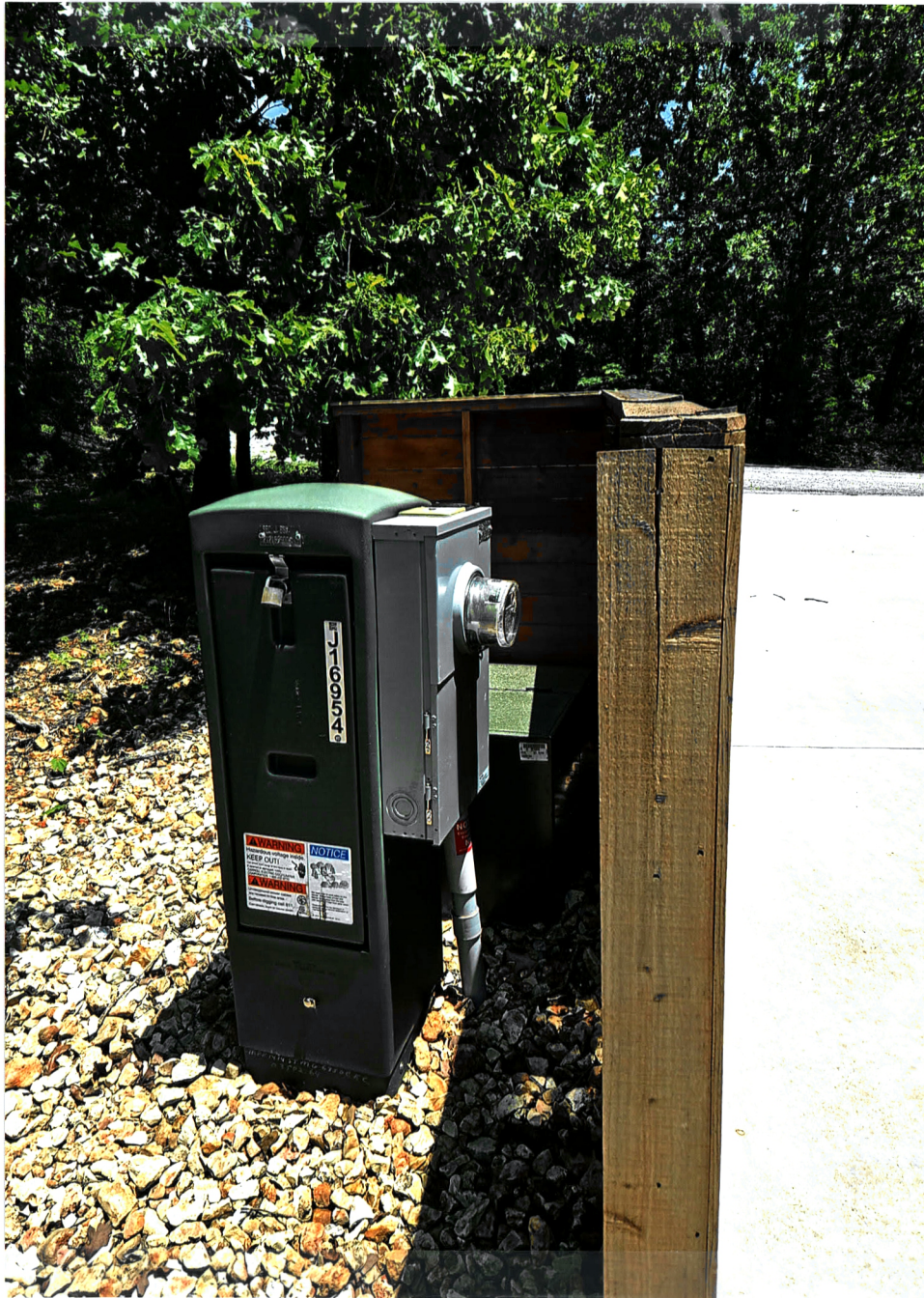
Tower with Safety Panel Screen
