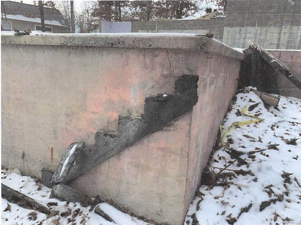
(Above / Below) Lower level CMU foundation (6'-0" Ht.) walls supporting backfilled slabs exhibit minor stains and drying shrinkage cracks that result from age and normal drying shrinkage. Walls can be cleaned with mild detergent and fractures repaired with epoxy adhesive.
