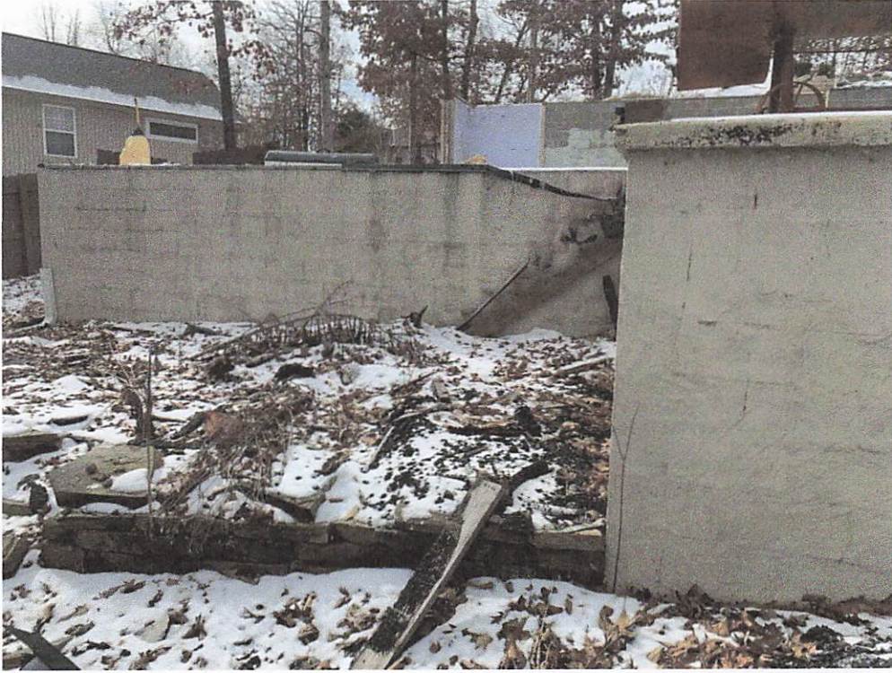
(Above / Below) Lower level CMU foundation (6'-0" Ht.) walls supporting backfilled slabs exhibit minor stains and drying shrinkage cracks that result from age and normal drying shrinkage. Walls can be cleaned with mild detergent and fractures repaired with epoxy adhesive.
